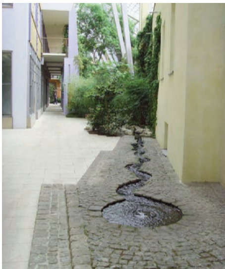
Creative internal rainwater use. Prisma, Nuremburg Architect: Joachim Eble, Photo: Janice Foster
