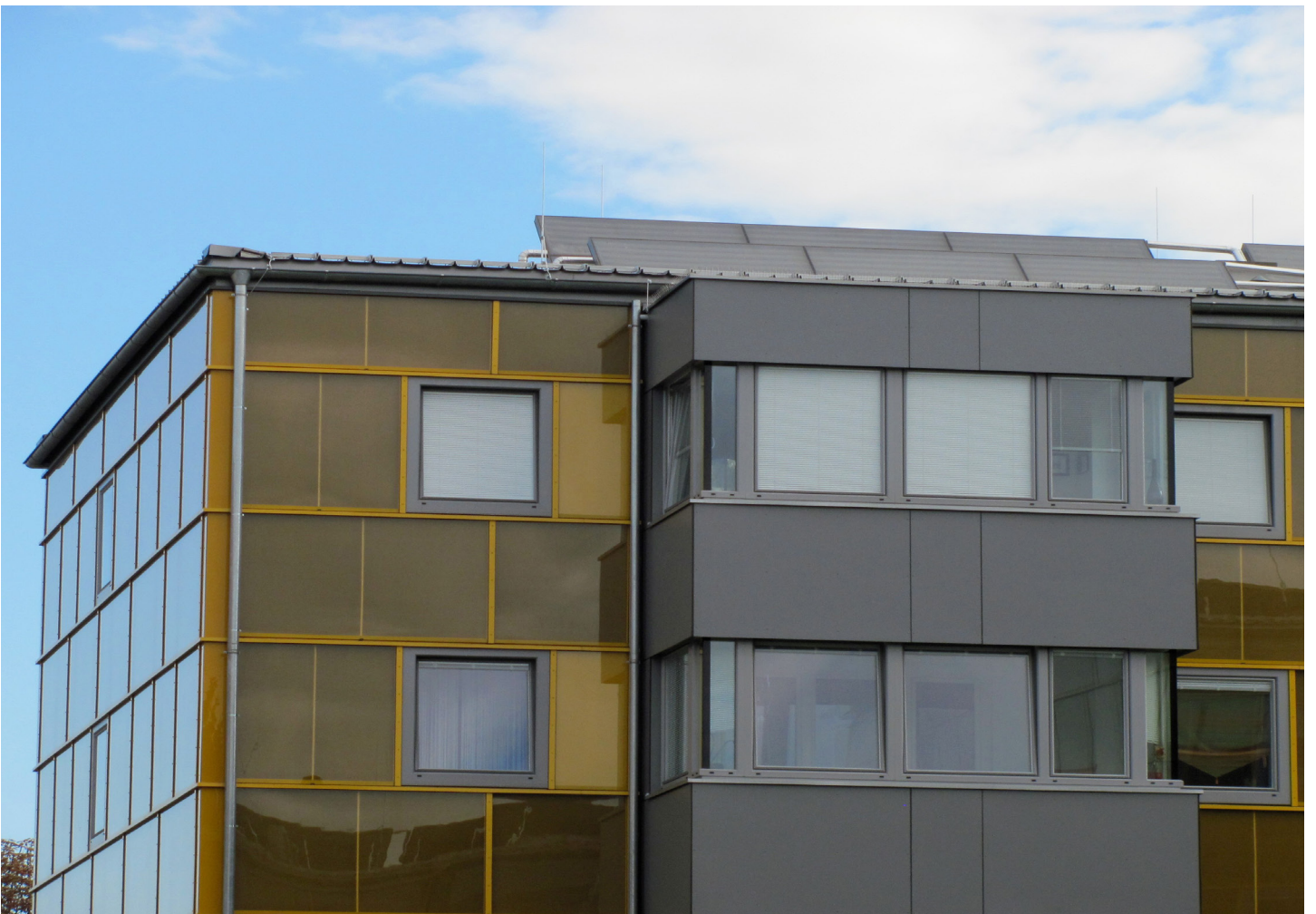
Image: Diesleweg 70 - decentralised MVHR panels (yellow) and sun spaces, SEDA Solar
