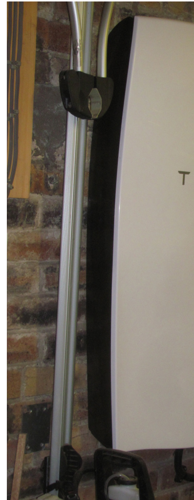
TESLA Powerwall, 6.4 kW discharge with nominal 8 kWh capacity Image Credit: Colin Porteous
