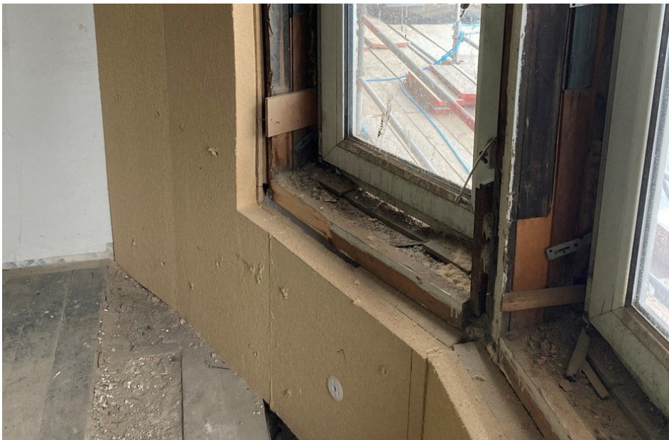
Above: Allows moisture in the wall to escape back into the room, especially when combined with good ventilation. Below: The use of hygroscopic insulation, like this wood fibre board on the inside of a stone wall. Image Credit: Chris Morgan
