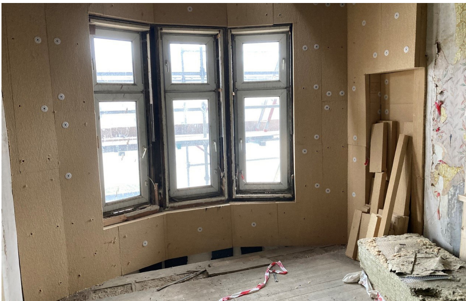
Above: Allows moisture in the wall to escape back into the room, especially when combined with good ventilation. Below: The use of hygroscopic insulation, like this wood fibre board on the inside of a stone wall. Image Credit: Chris Morgan
