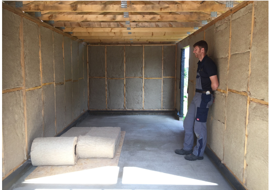
Sisaltech garage application
