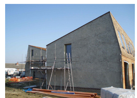
Rachel Bevan Architects - Elmswell hemp housing in progress
