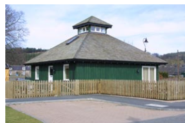
Design for deconstruction is most effective when it allows for maximum flexibility of spatial configuration. Source: F. Stevenson
