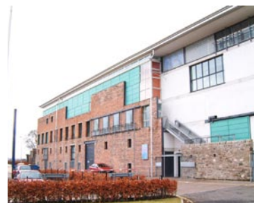
Dundee Contemporary Arts Centre. Visible re-use of existing local building fabric preserves historic understanding and maintaining a link with the past. Source: N. Verow
