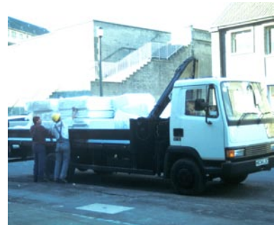
Obtain re-used materials locally in order to reduce transportation impacts. Source: F. Stevenson
