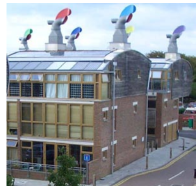
Using reclaimed timber at BedZed, made an overall cost saving. Source: F Stevenson
