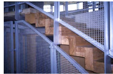
Re-used railway sleepers forming new stairs. Source: F. Stevenson
