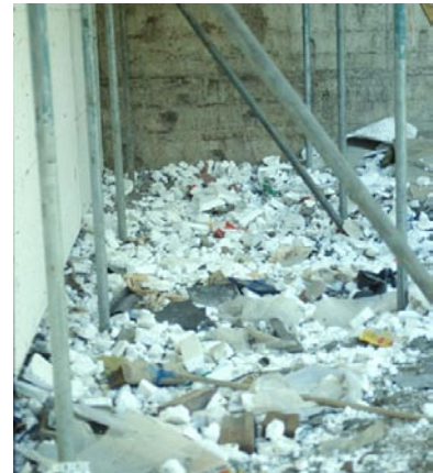
Unnecessary construction waste can be prevented through re-use. Source: F. Stevenson
